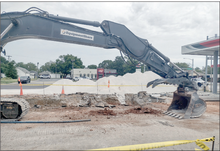
Old 5,000-gallon storage tanks have been removed from Rapid Roberts location in Monett, with new ones scheduled to take their place. Sheila Harris/sheilaharrisads@gmail.com
