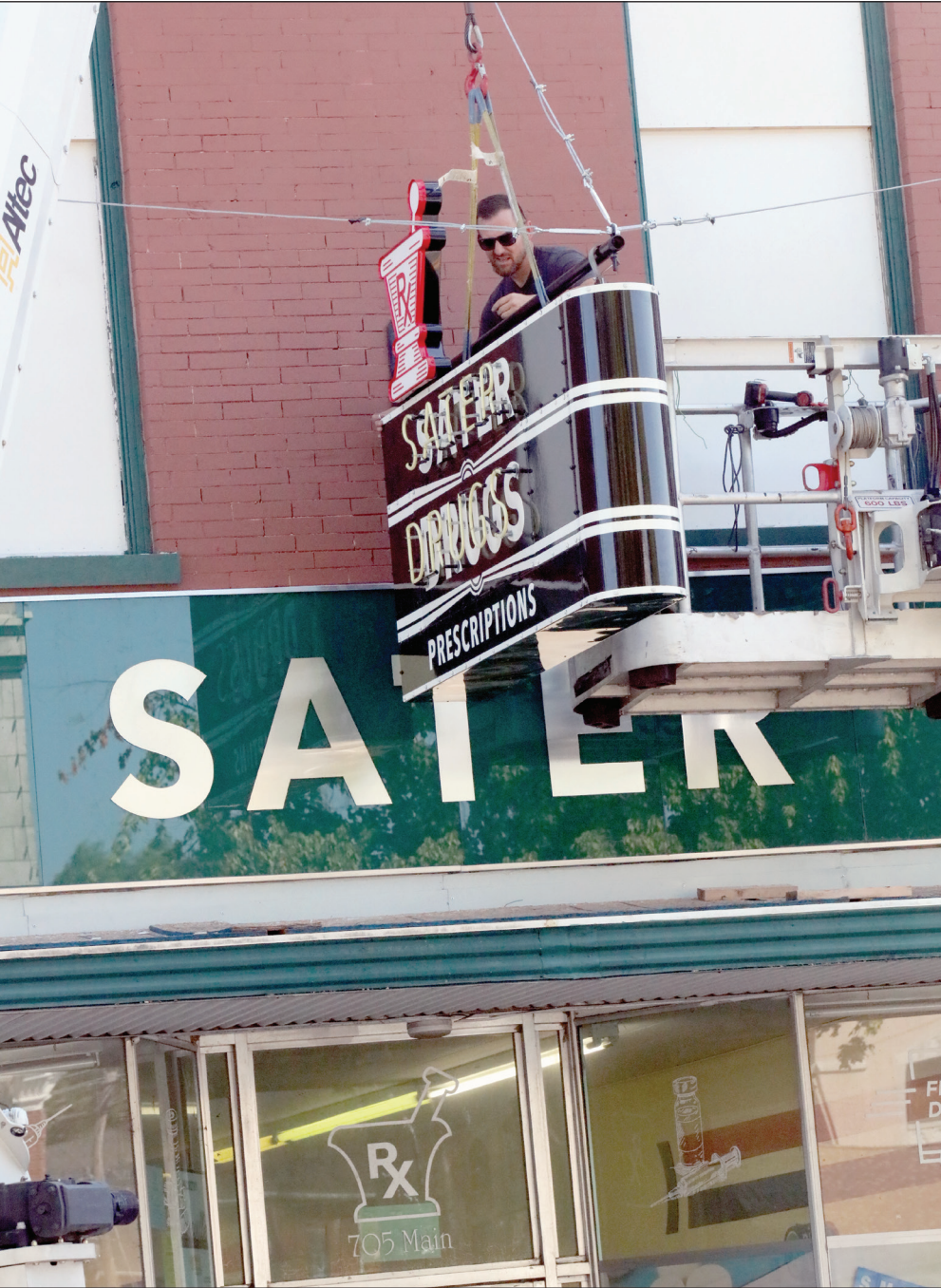
Jeremy Wilson, with Tulsa-based Crown Neon Signs, installs the new signage at Sater Pharmacy, meant to mimic historic neon signage on the Cassville square. Funding for the project was provided by the Community Foundation of the Ozarks' Cassville Downtown Restoration Fund. Kyle Troutman/ktroutman@cassville-democrat.com
