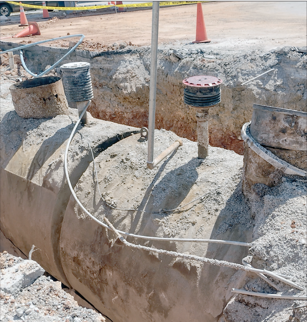
Two, 10,000-gallon, fuel-storage tanks, as well as gas distribution lines, will be replaced at Rapid Roberts, in Monett, after approximately 50 gallons of gasoline was released into the ground from a line to one of the gas dispensers on June 17. The fuel storage tanks have been in the ground since the mid-1980s, said Rapid Roberts' director of compliance, Steve Makoski. Sheila Harris/sheilaharrisads@gmail.com
