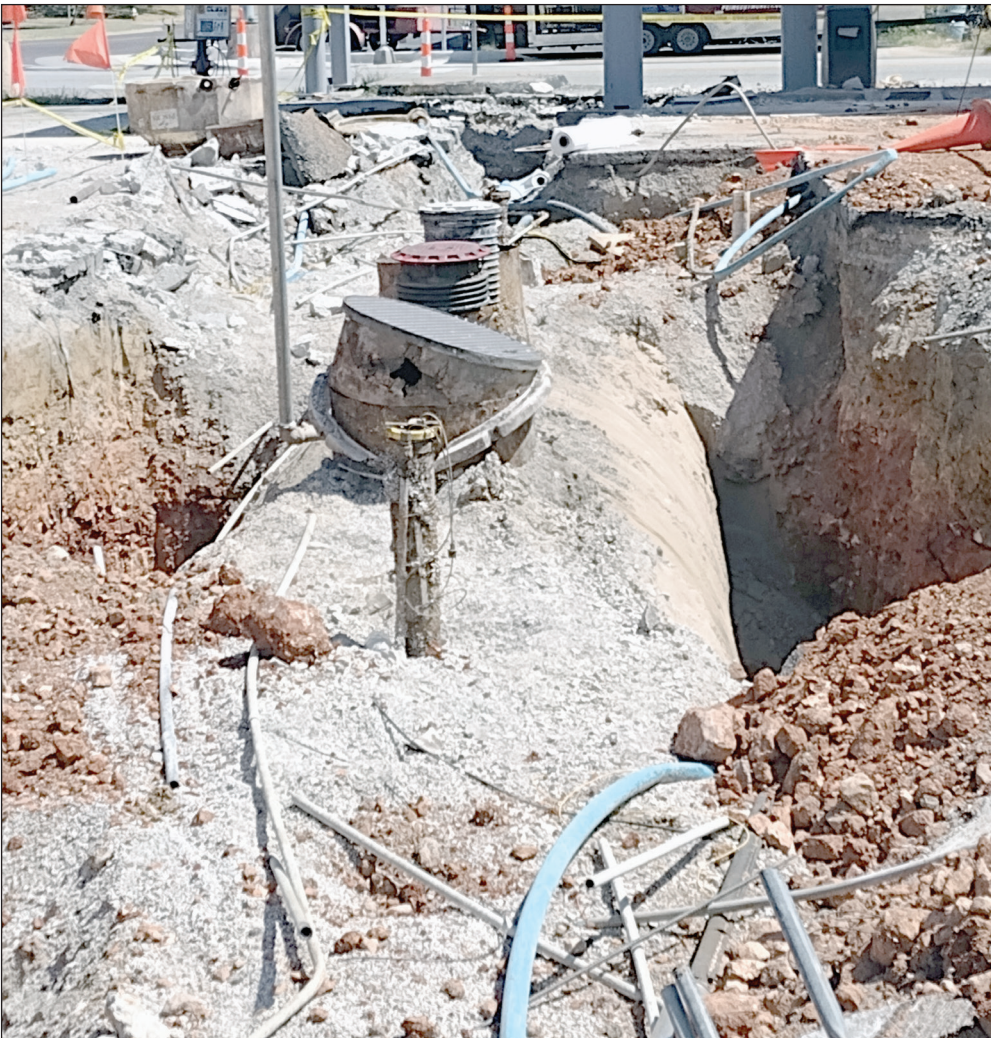
Two, 10,000-gallon, fuel-storage tanks, as well as gas distribution lines, will be replaced at Rapid Roberts, in Monett, after approximately 50 gallons of gasoline was released into the ground from a line to one of the gas dispensers on June 17. The fuel storage tanks have been in the ground since the mid-1980s, said Rapid Roberts' director of compliance, Steve Makoski. Sheila Harris/sheilaharrisads@gmail.com
