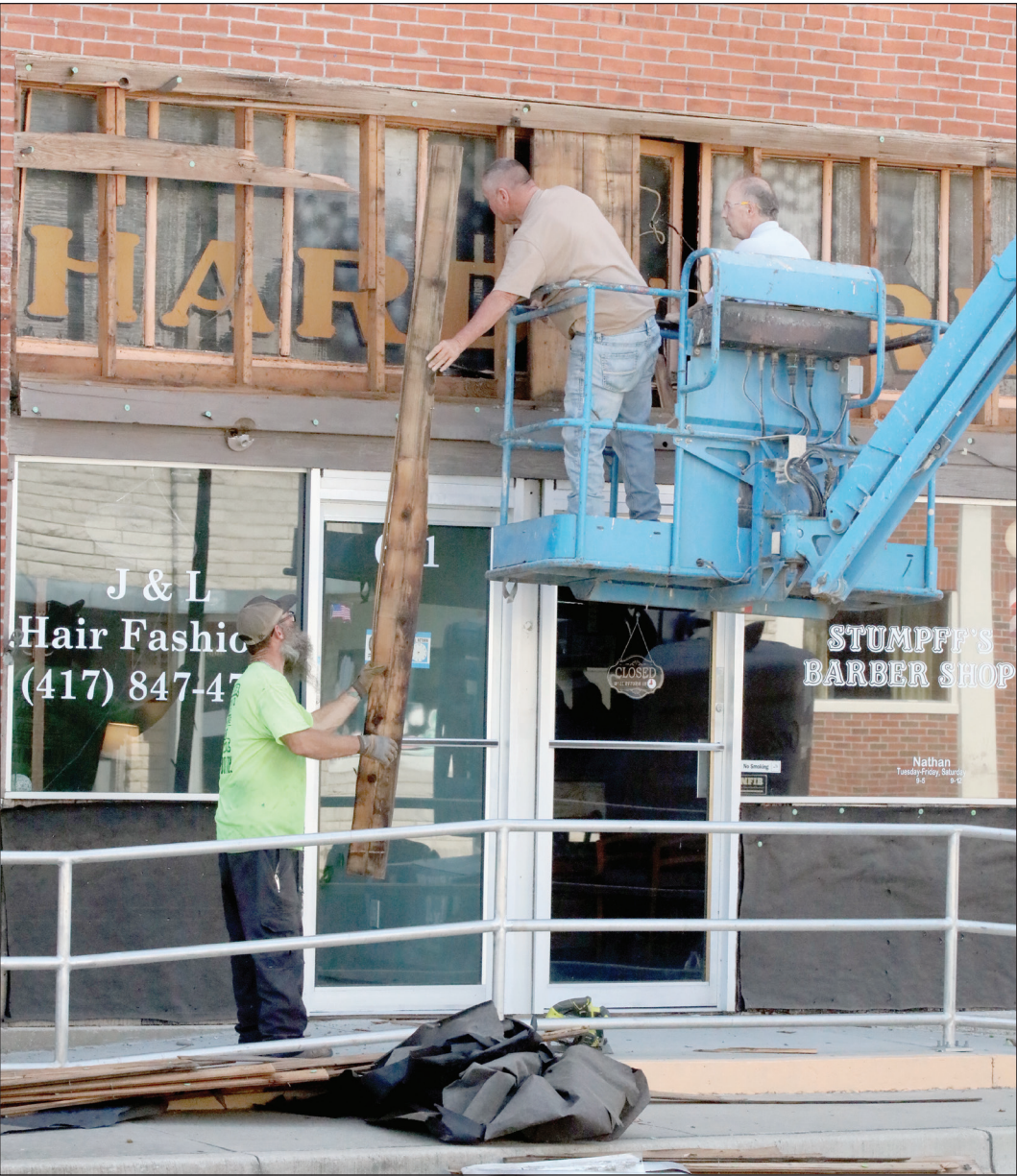
Carl Schell, center, with Carl Schell Construction, hands down a piece of plywood to Frank Diaz while working on the facade of Zachary Fields' building on Main Street on Monday. Under the wood was a "Hardware" sign made of single-pane glass. The former Haddock & Meador Hardware Store operated through the 1970s. Now, the building houses J&L Hair Fashion salon and Stumpff Barbershop. Kyle Troutman/ktROUTMAN@cassville-democrat.com
