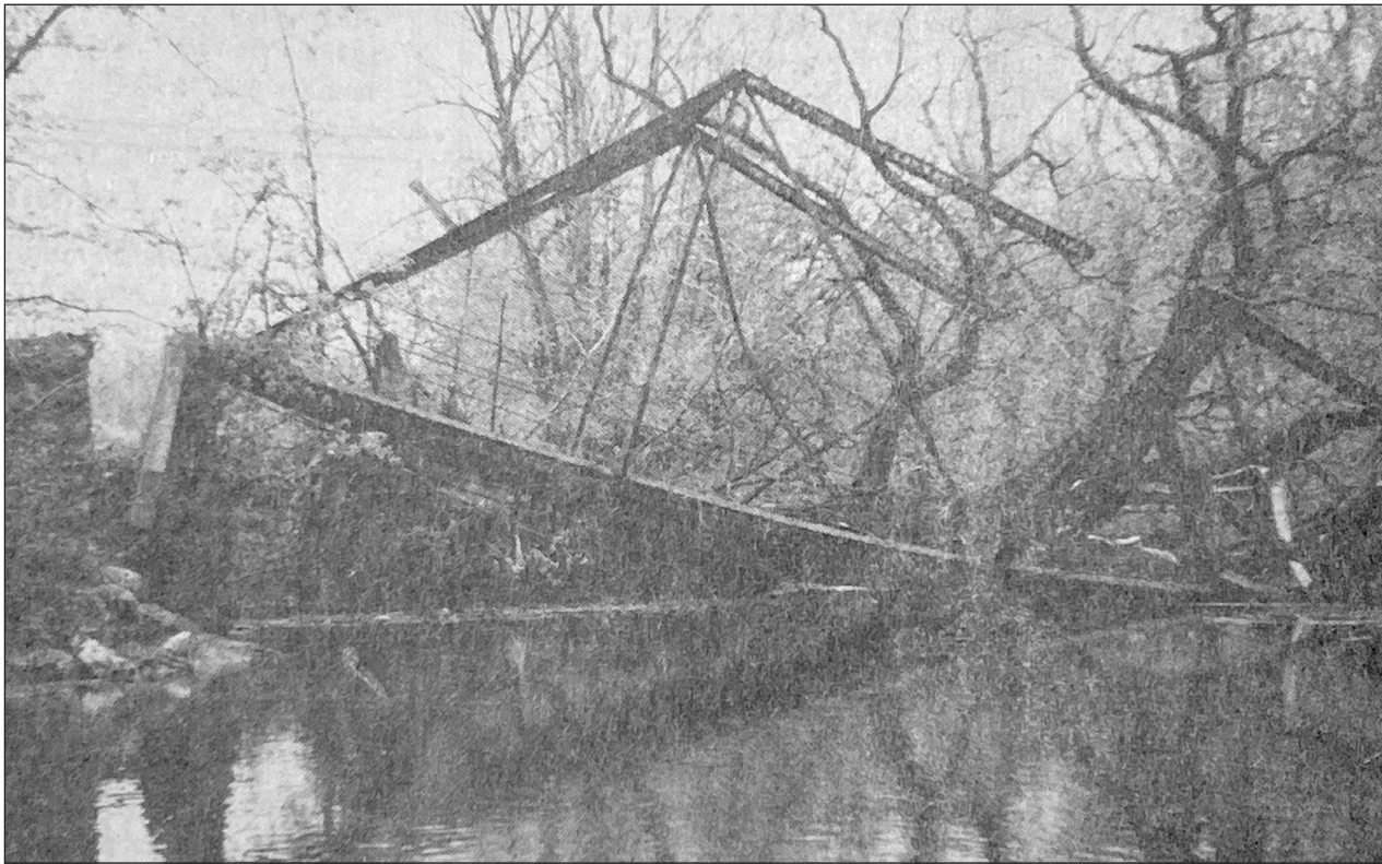
30 YEARS AGO: STORMY WEATHER — One of the largest casualties of Sunday's storm was the destruction of a bridge over Flat Creek at Stubblefield Crossing. High winds blew a massive oak tree onto the bridge, knocking it down into the creek and demolishing it. Presiding Commissioner Cherry Warren stated he did not know when funds could be secured to replace the bridge. Democrat file photo
