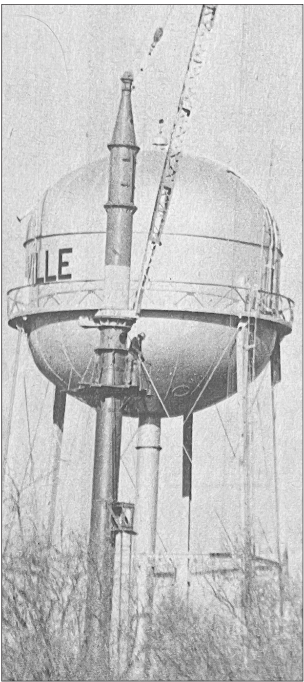
50 YEARS AGO: AND SOON THERE WILL BE TWO — This telephoto shows work in progress in putting a new 150,000-gallon water tower in place for Cassville. The tower will be used by contractors to hoist sections of the water storage facility into place. To give some size of the project, a crewman is standing on a tower platform with the bottom of the present tower in the background. Completion of the project will finish a water improvement program that included a new well at the FASCO Plant and line extension in the south part of town. The new tower is located directly south of the present tank. Contracts on the entire project were funded by a $270,000 bond issue passed in May 1974.
