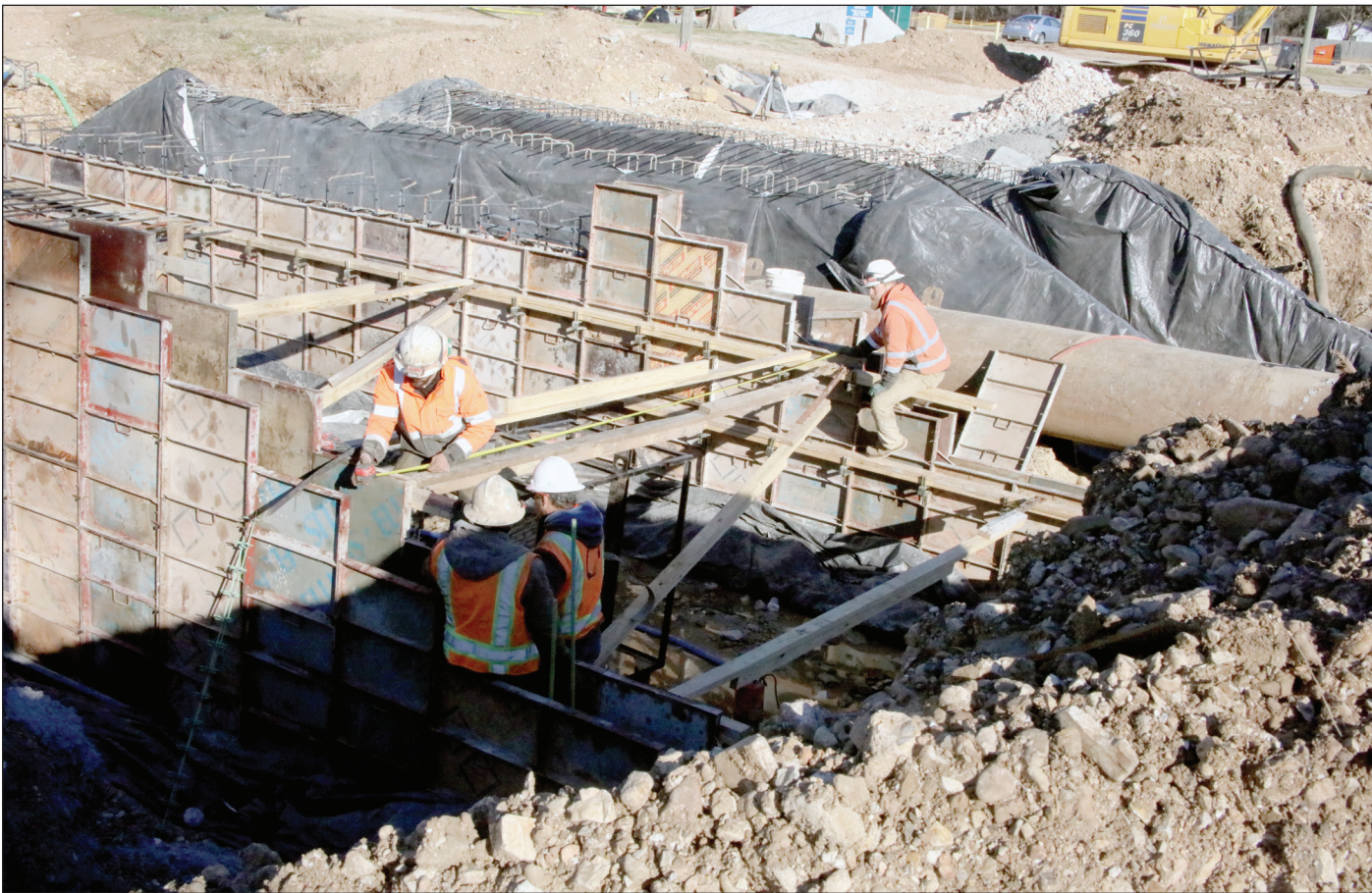
Construction crews working on the 7th Street Bridge project install culvert walls for the incoming bridge. Hartman and Company was awarded the bid at $738,000, and the new 15-foot triple-span reinforced concrete box bridge over Flat Creek will replace the low-water crossing damaged beyond repair by flash flooding in 2017. The project is set to be completed by May, complete with a vehicular crossing and sidewalk pedestrian crossing, and it may open sooner to allow for travel prior to being paved. Kyle Troutman/kt troutman@cassville-democrat.com
